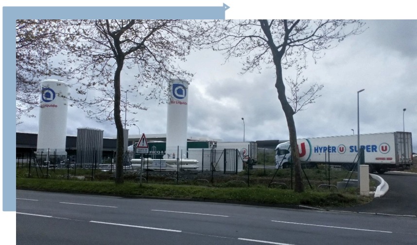
Station Air Liquide à Ploufragan (22) / Mixenn
