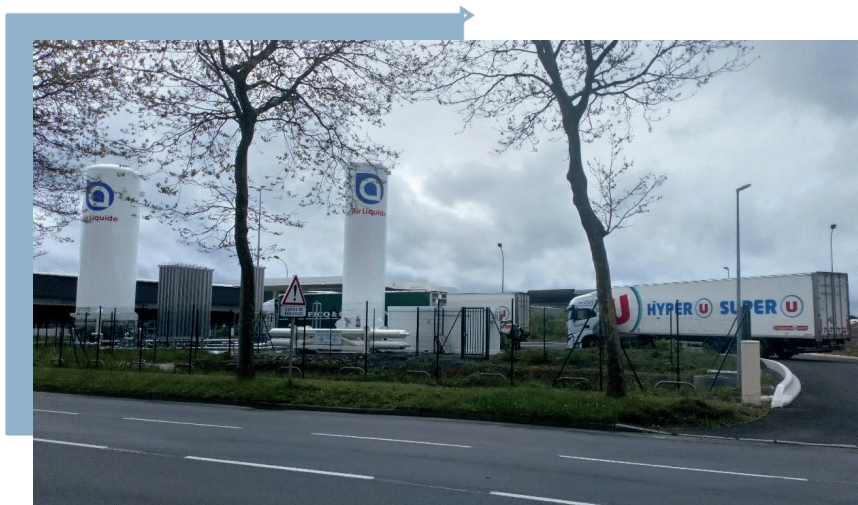
Station Air Liquide à Ploufragan (22) / Mixenn
